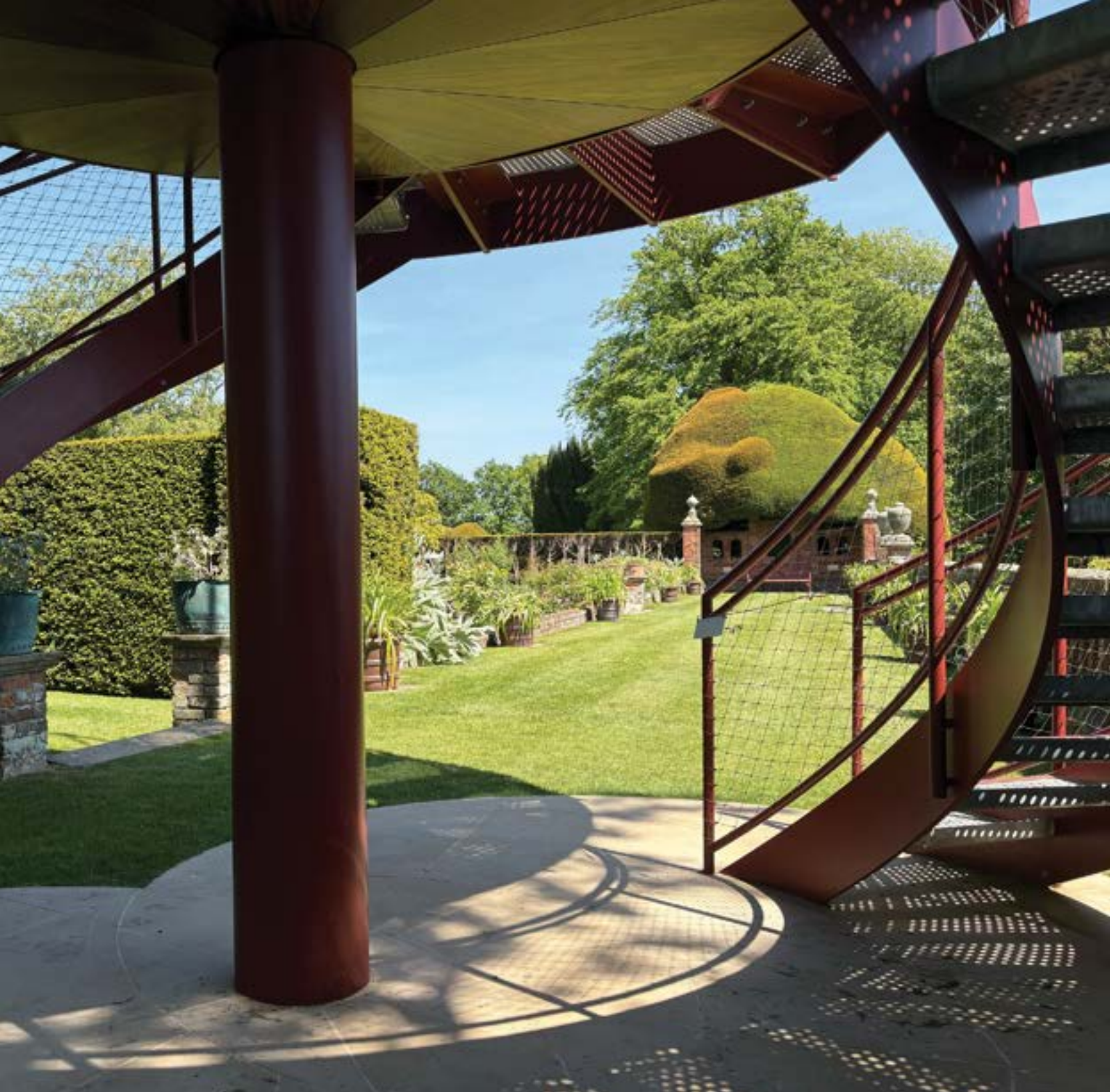
Fig 2: The ground level of the tower is embraced by the two curving stairs. A single, central post supports the whole structure
